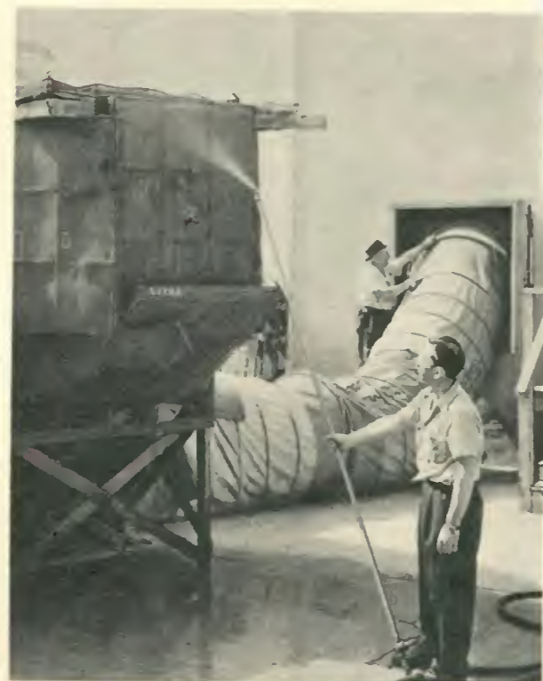
IN SPITE of the cooling machines employed to give some relief on the stages, sweltering weather aided by heat from klieg lights still made acting uncomfortable on "The Little Foxes" set
